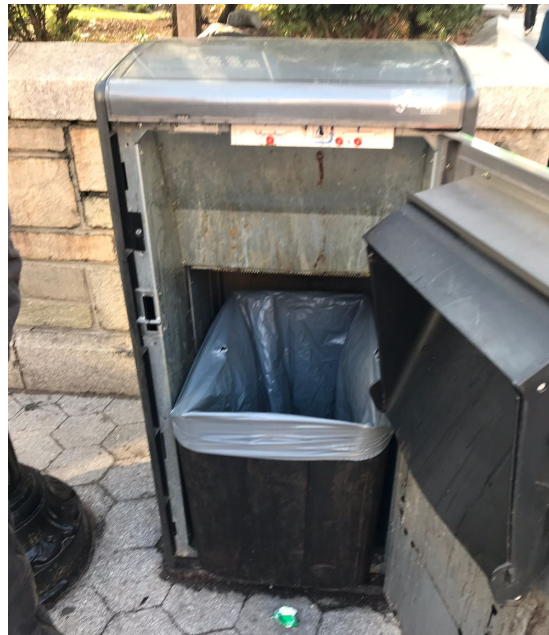
Figure 4: Inside a Bigbelly Waste Bin
